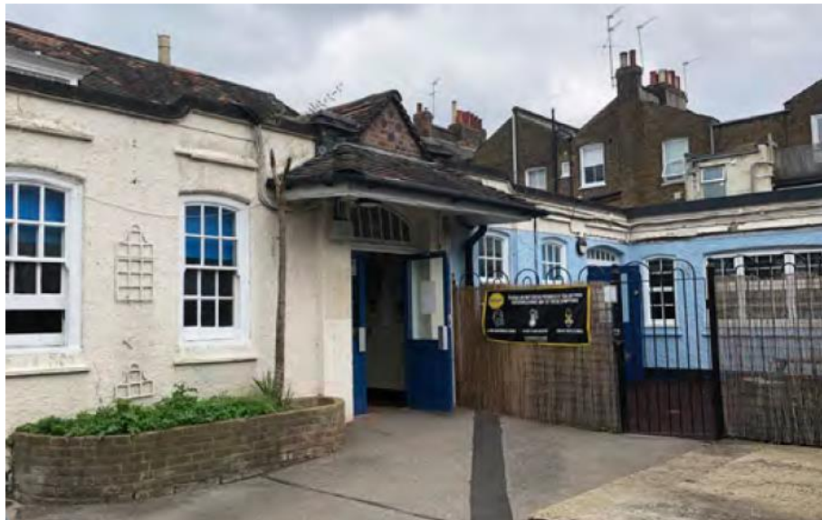
Figure 7 – View of main entrance to school building
